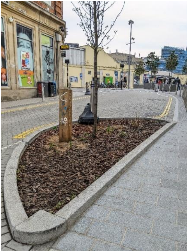
Figure 7.2 Rainwater Garden, Chertsey Road
